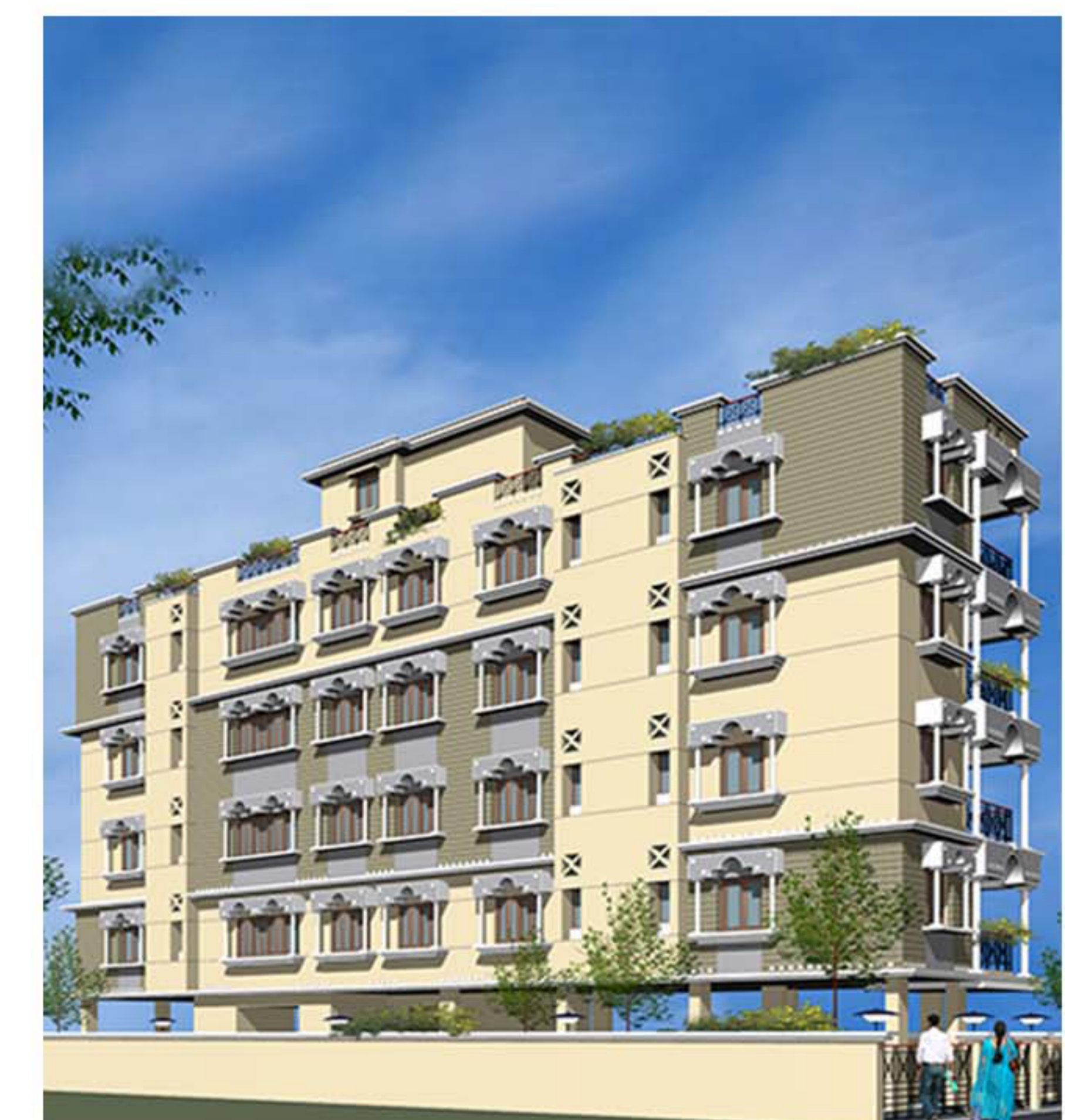
G+IV STORIED RESIDENTIAL BUILDING H.M.SARANI
